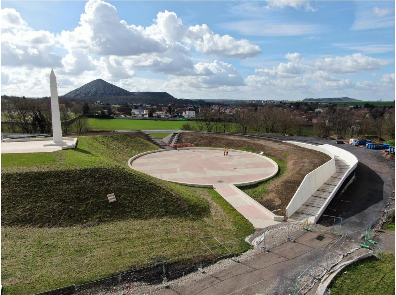
*A drone photograph of the construction of the Frederick Lee walkway, which has a trench and a bridge, thereby making it NATO's most expensive walkway! This allows the uphill gradient to satisfy disabled access to the obelisk.*
