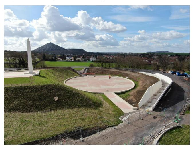
A drone photograph of the construction of the Frederick Lee walkway, which has a trench and a bridge, thereby making it NATO's most expensive walkway! This allows the uphill gradient to satisfy disabled access to the obelisk.
